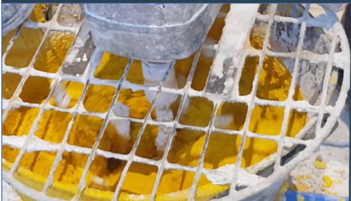
Material is mixed and ready to be poured into respective areas
