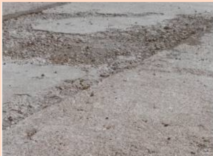
Concrete Spalling
