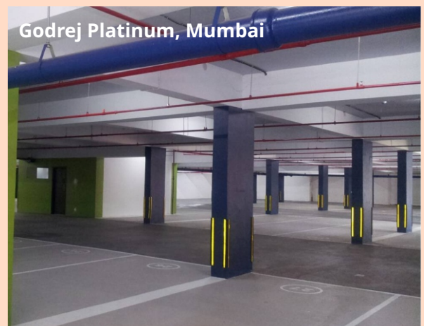
Details of Floor for Parking Deck for exterior areas 1.5 to 2 mm PU self-leveling flooring system with textured topping
