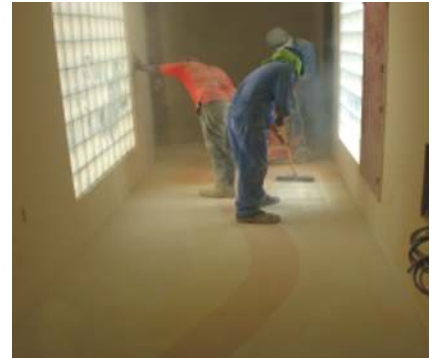
Cured epoxy terrazzo is ground and polished
