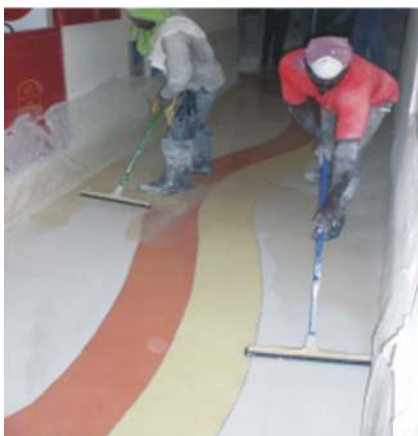
Grouting, Washing & Cleaning
