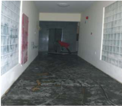
Epoxy primer applied surface with the pattern set on the floor
