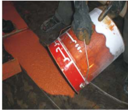
Epoxy terrazzo mix is poured into the respective patterns
